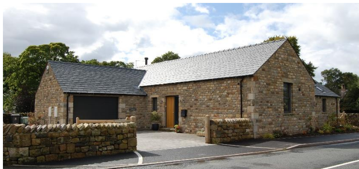
Wenningdale - An example of recent residential development
