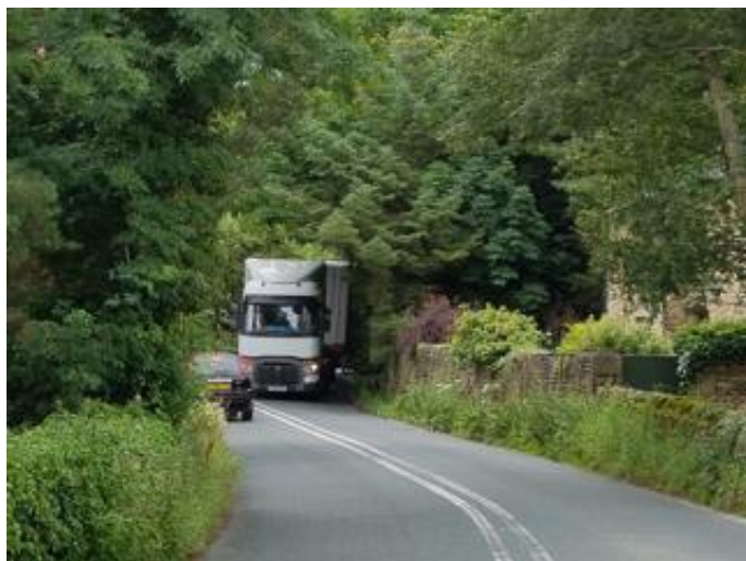
The lack of a footway east of the village
